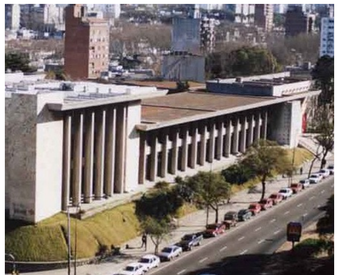
Faculty of Architecture, Design and Urbanism (University of the Republic - Uruguay), designed by Fresnedo Siri and Muccinelli in 1946.
